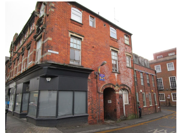
Plate 67 No. 29 Corporation St is an example of an architecturally interesting building that is suffering from under use and inappropriate alterations such as the replacement of historic windows with Upvc frames
