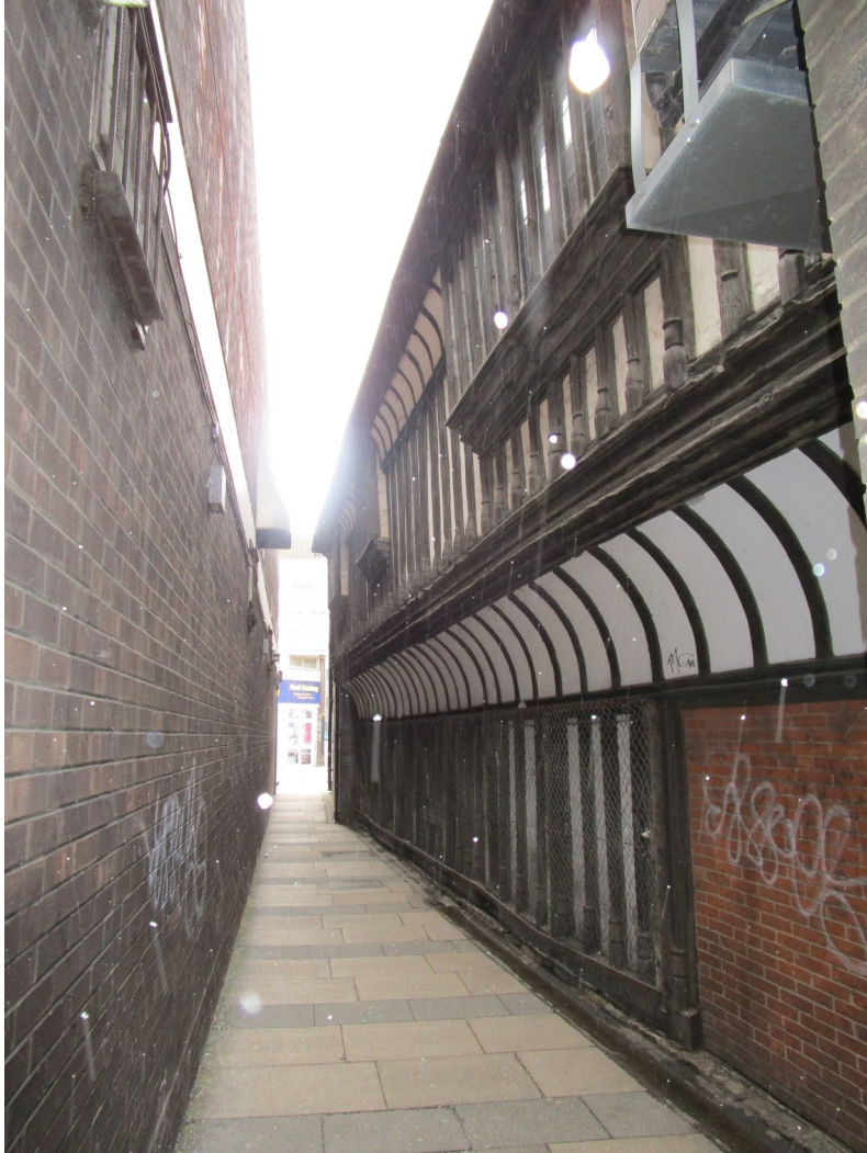
Plate 71 Arkills Yard, No. 353 High St, modern development has been built up against this historic façade.
