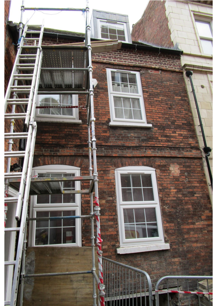
Plate 72 Building to rear No. 47 Silver St, replacement of historic windows with Upvc replacements threatens the conservation area.
