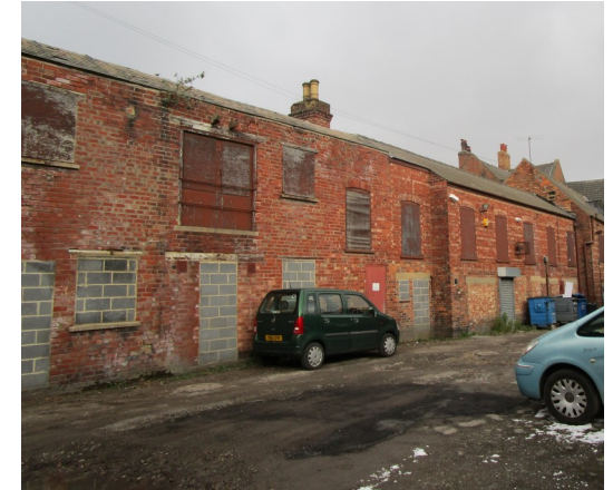
Plate 29 Former industrial buildings at the rear of No. 172 High Street
