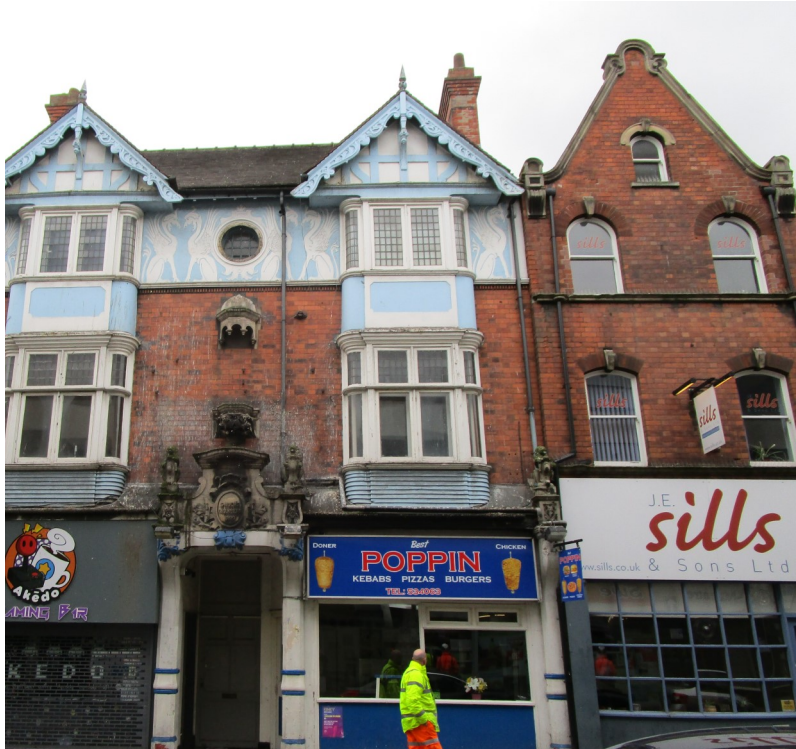
Plate 57 St Hughes Chambers, Corporation St is a Grade II listed office or lawyers building and dates from 1899. It has distinctive carved barge boards and griffins formed in relief by pargeeting on the 2 nd floor.
