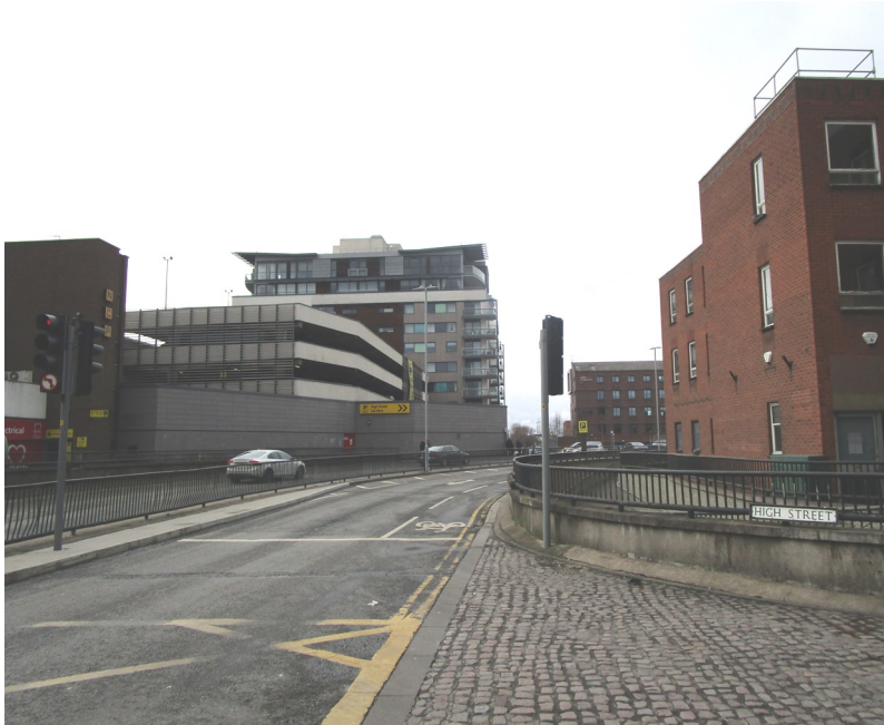
Plate 69 The construction of Wigford way has cut through the historic burgrave plot development here and created an open, highway-dominated space at odds with the historic character here.
