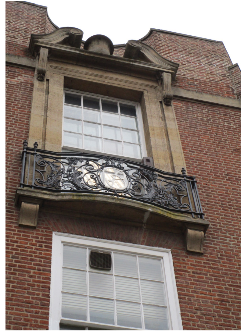
Plate 39 No. 280-281 High St and 1-3 Clasketgate, the former Boots department store and job centre has a splayed corner with a stone window surround with an open pediment and urn, and juliet balcony with the Boots corporate lettering.
