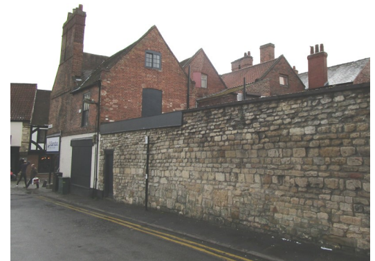
Plate 43 Boundary wall to rear No. 265 High St, an example of a stone boundary wall along an historic burgage plot boundary.
