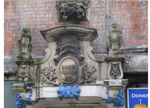
Plate 66 Defective rainwater goods are threatening this building, St Hugh's Chamber, Corporation St
