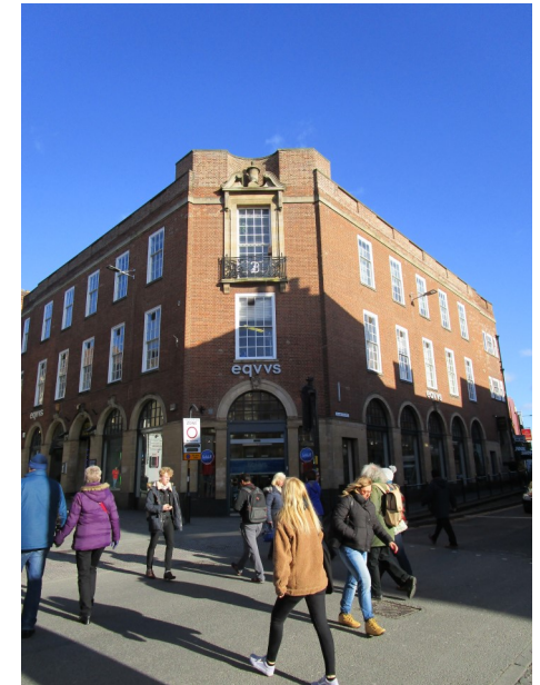
Plate 16 No. 280-281 High Street and 1-3 Clasketgate, Former Boots Department Store and Job Centre
